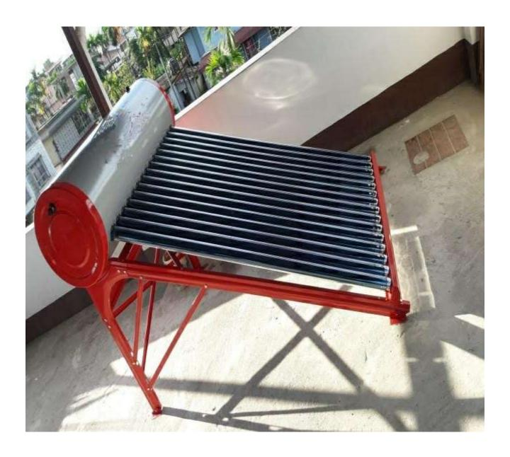
01. Supply and installation of solar water heating system (200LPD) [SOLAR WATER HEATER] with the existing soft water source [including plumbing work up to 30 feet]
